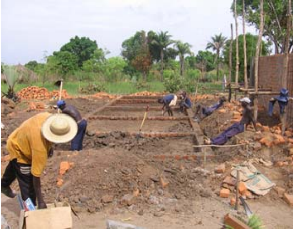
Foundation - Office Building (Left) Preparing for Ceiling of Training Hall (Right)
